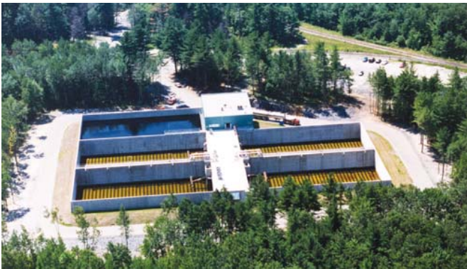
Secondary effluent treatment system Brompton, Québec
