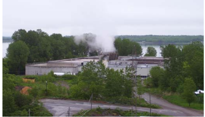
Secondary effluent treatment system Kruger Wayagamack, Trois-Rivières, Québec
